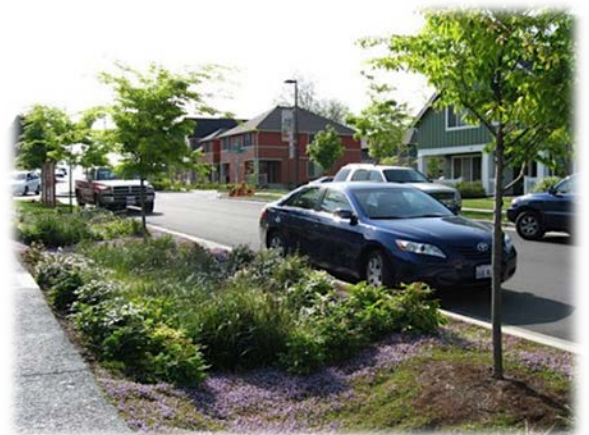
Water from hard surfaces can be directed into swales to fully irrigate native and climate appropriate plants.
